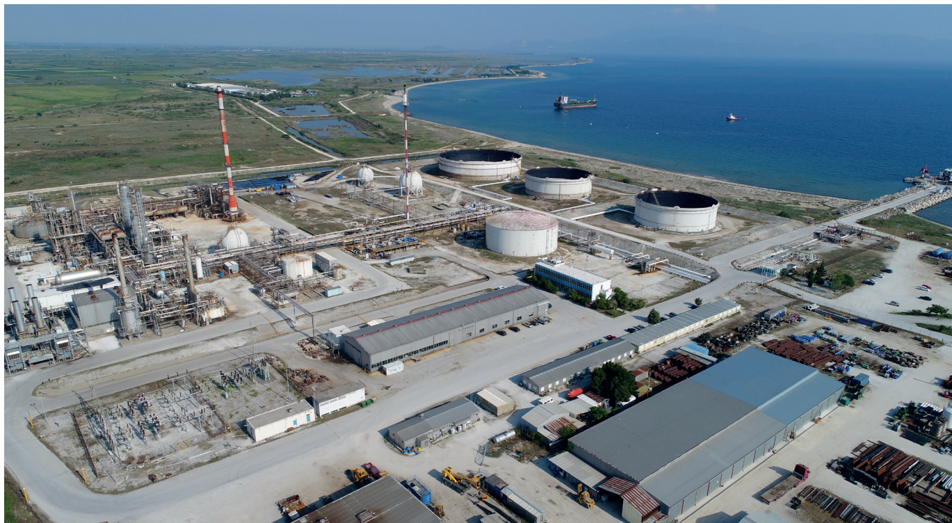
Work in progress: Greece's energy sector is expanding, with a focus on E&P
